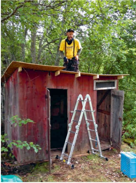
Anders reparerar Gunbos uthus
